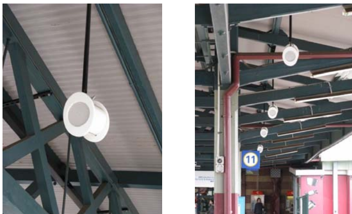
Figure 15: Photographs of steered time sequenced system as installed at Sydney Central Station
