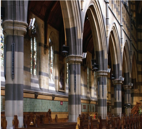
The AT Line arrays installed on the church columns...
