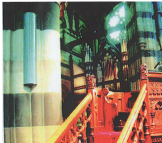
Acoustic Technologies ALA07C near the pulpit
