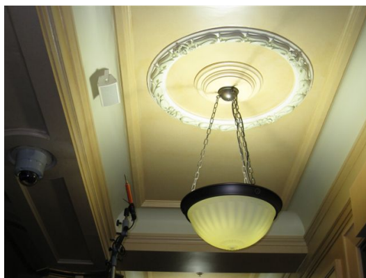
Figure 6: Cornice Type Loudspeaker taking advantage of bulkhead shielding
