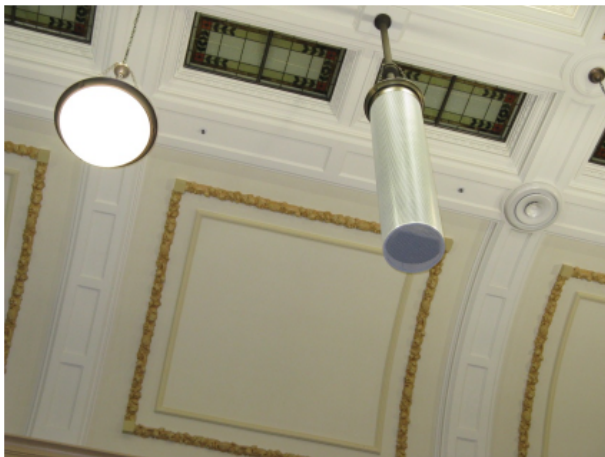
Figure 2: "Kiwi-tube" in situ with perforated metal shroud
