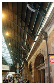
Eight arrays of 12-element Omniline loudspeaker elements cover the Concourse
