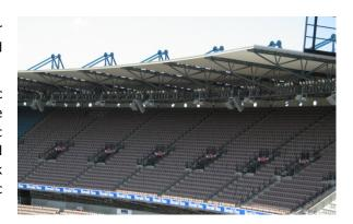
Among the benefits that Acoustic Directions brought to this project was a steered bass loudspeaker array whose unusual radiation pattern substantially overcame the wide variation in the distance from listener seats to the loudspeakers, enabling a much more consistent distribution of sound at low frequencies.
