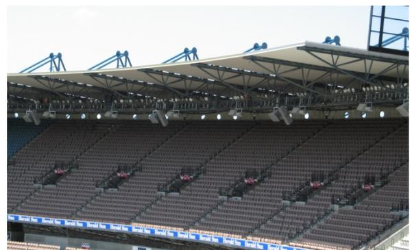
Among the benefits that Acoustic Directions brought to this project was a steered bass loudspeaker array whose unusual radiation pattern substantially overcame the wide variation in the distance from listener seats to the loudspeakers, enabling a much more consistent distribution of sound at low frequencies.
